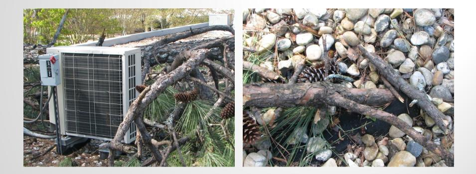
Debris on roof from over-hanging limbs can cause the drains to clog and allow water into the building depending on roof design. Roofs are cleaned on a monthly PM (Preventive Maintenance).
